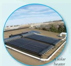
Solar heaters change solar energy into heat energy that is used for warming and heating of water.
